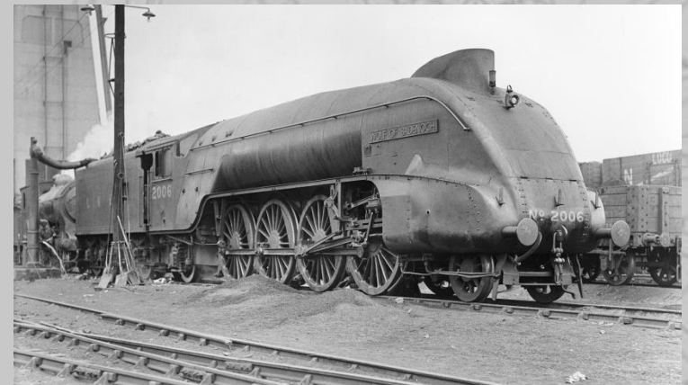
No. 2006 Wolf of Badenoch - longer combustion chamber in firebox to aid combustion prototype for Tornado's boiler
