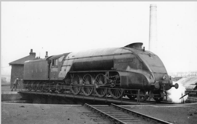
No. 2005 Thane of Fife - single (non-Kylchap) chimney
