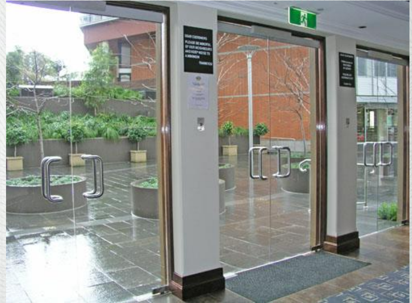
1 set of frameless glass doors - 350 Pa on doors = approximately 80 lb force to open each door
