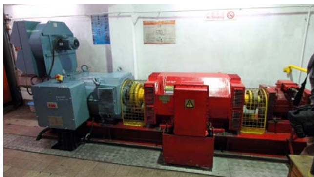
560 kW a.c. motor (blue; left) coupled with 545 kW d.c. generator (red; right) inside Haulage Room [Benny S.Y. Sit]
