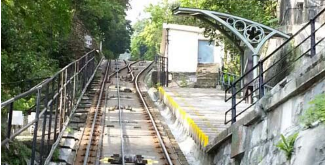
Passing Loop, outside May Road stop (left hill-side for “White Tramcar”) [W.H. Tsang]
