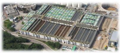
to collect foul gas from the covered tanks, channels and chambers and treatment of foul gas by 'Biotrickling Filter' technology before discharge into open air.
