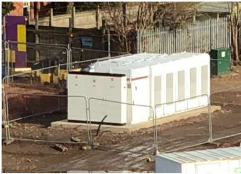
Tesla 2.1MWh Battery - 500kW inverter
