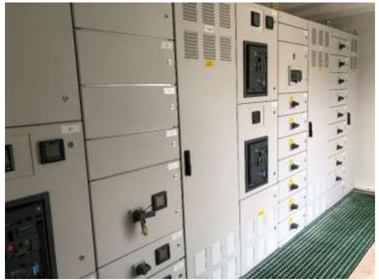
Low Voltage Distribution Panels
