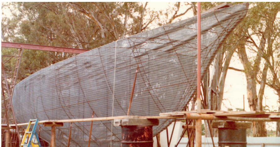
Athena in skeletal form, with some mesh and longitudinal reinforcing.
